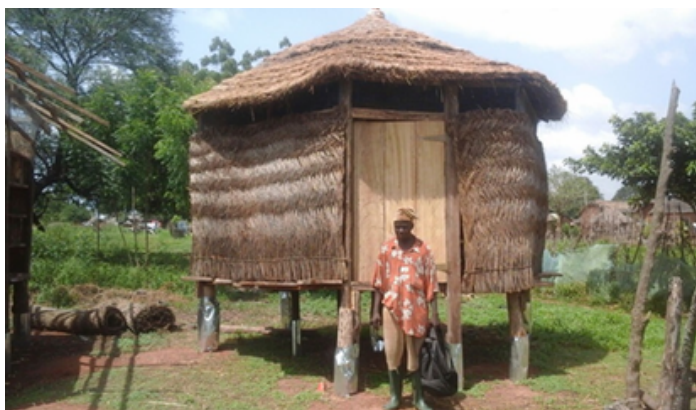
Plate 9: Yam storage facility using thatch wall
